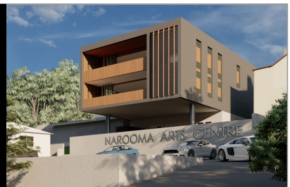
Proposed Narooma Arts & Community Centre from the rear (Garvan Street), with Kinema, right, and Studios to the left. Source ClarkeKeller
