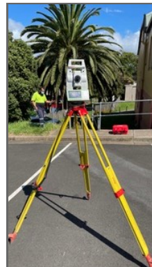
More survey work is done
